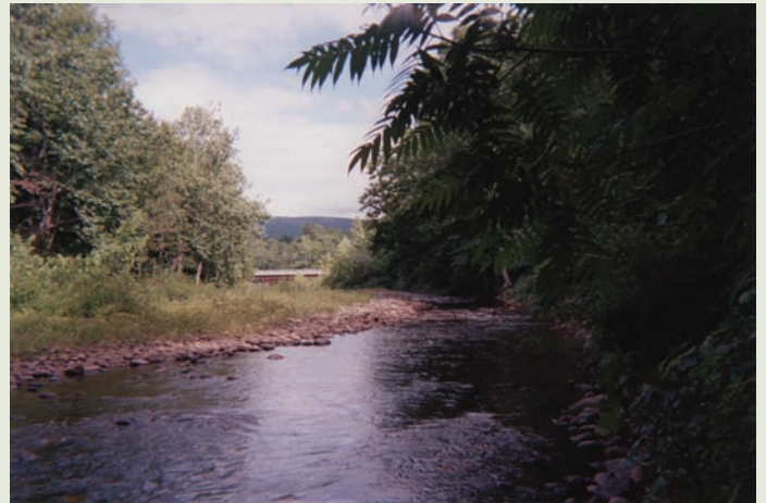
Mass bank failure at confluence of Roaring Branch & Batten Kill. (Top) Looking upstream toward the Route 7A bridge. (Bottom)
