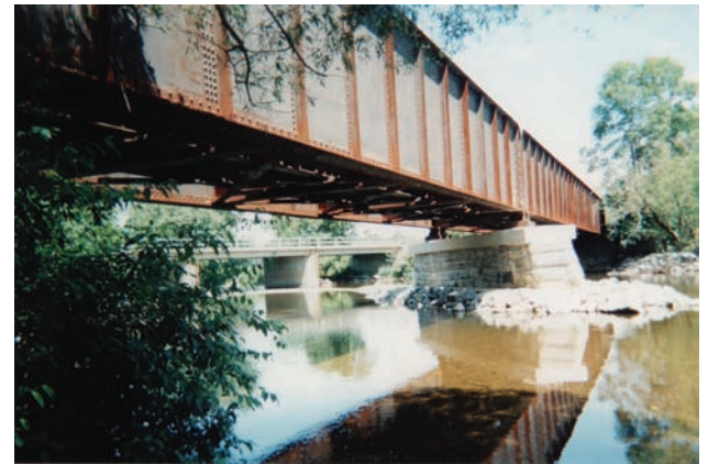
The reconstructed RR bridge in Shushan NY.
