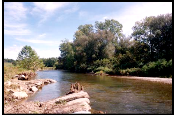
Rock vanes angled upstream to restore a meander and improve river dynamics at Foster Farm in Shushan, NY. Vanes with the open end upstream direct the force of the current back to the center and build up sediment deposits behind them.
