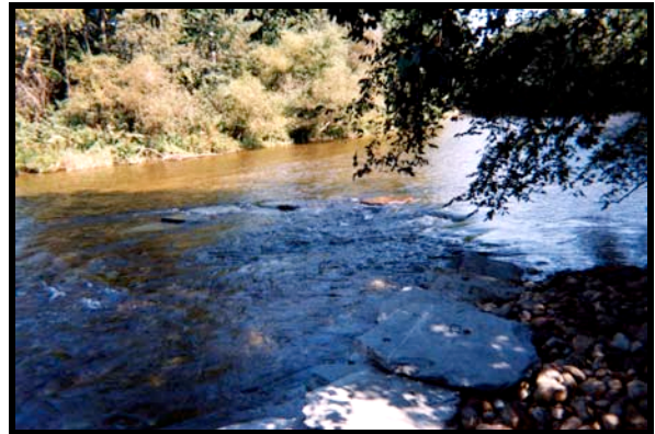
Looking upstream at stone J-hook to improve river dynamics and stabilize bank at Hibrow Farms, Salem, NY. [NY photos by C. Browning.]
