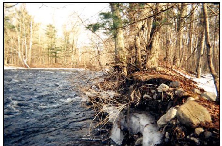
Photo is looking upstream along Roaring Branch berm in high water. Removal of berm would allow access to flood plain at right.
