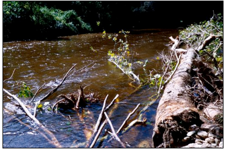
New large woody debris structure provides cover and shelter for trout along Twin Rivers Extension project.
