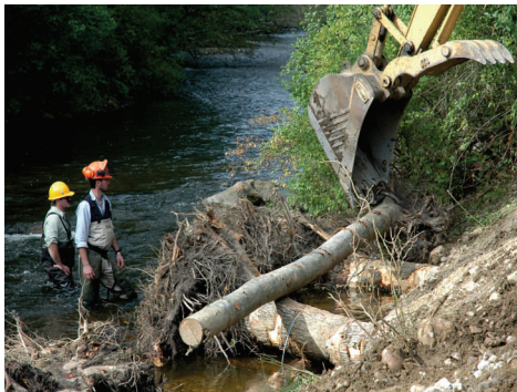
Fish cover habitat construction in Manchester.
