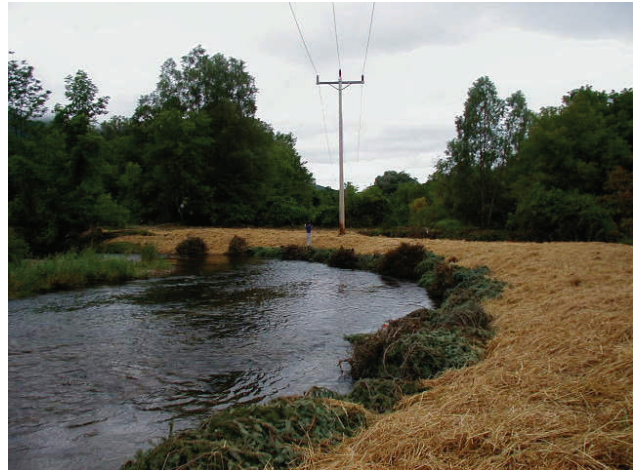
Tree revetments at Wilburs' Bridge site
